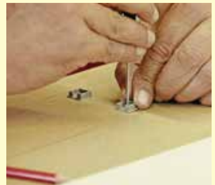
3. At the joins of the rail routes, floor slabs for the pillars are screwed on.
